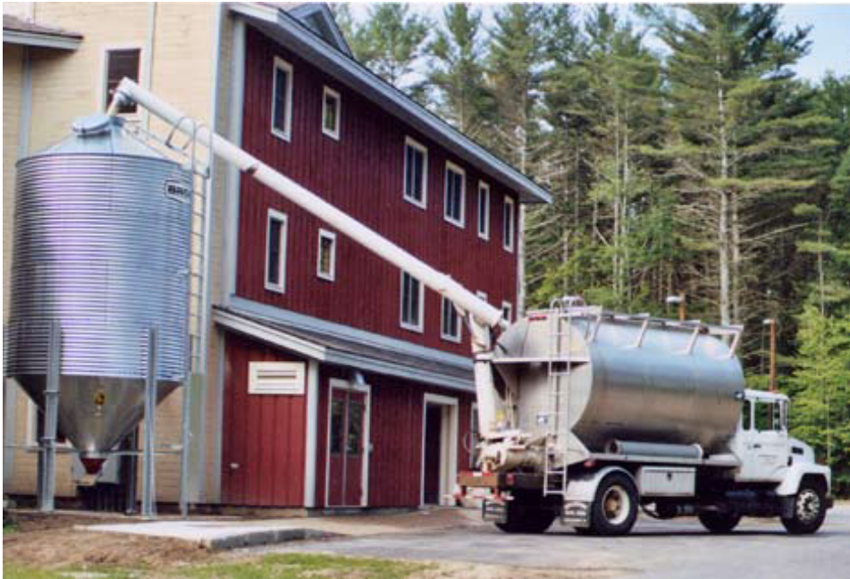
Figure 6 Bulk Pellet Storage and Delivery 9
