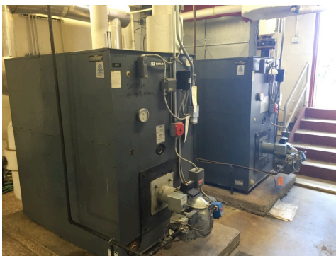
Figure 2 Middle/High School 2001 2 - HB Smith Boilers on left, Burnham boiler on right
